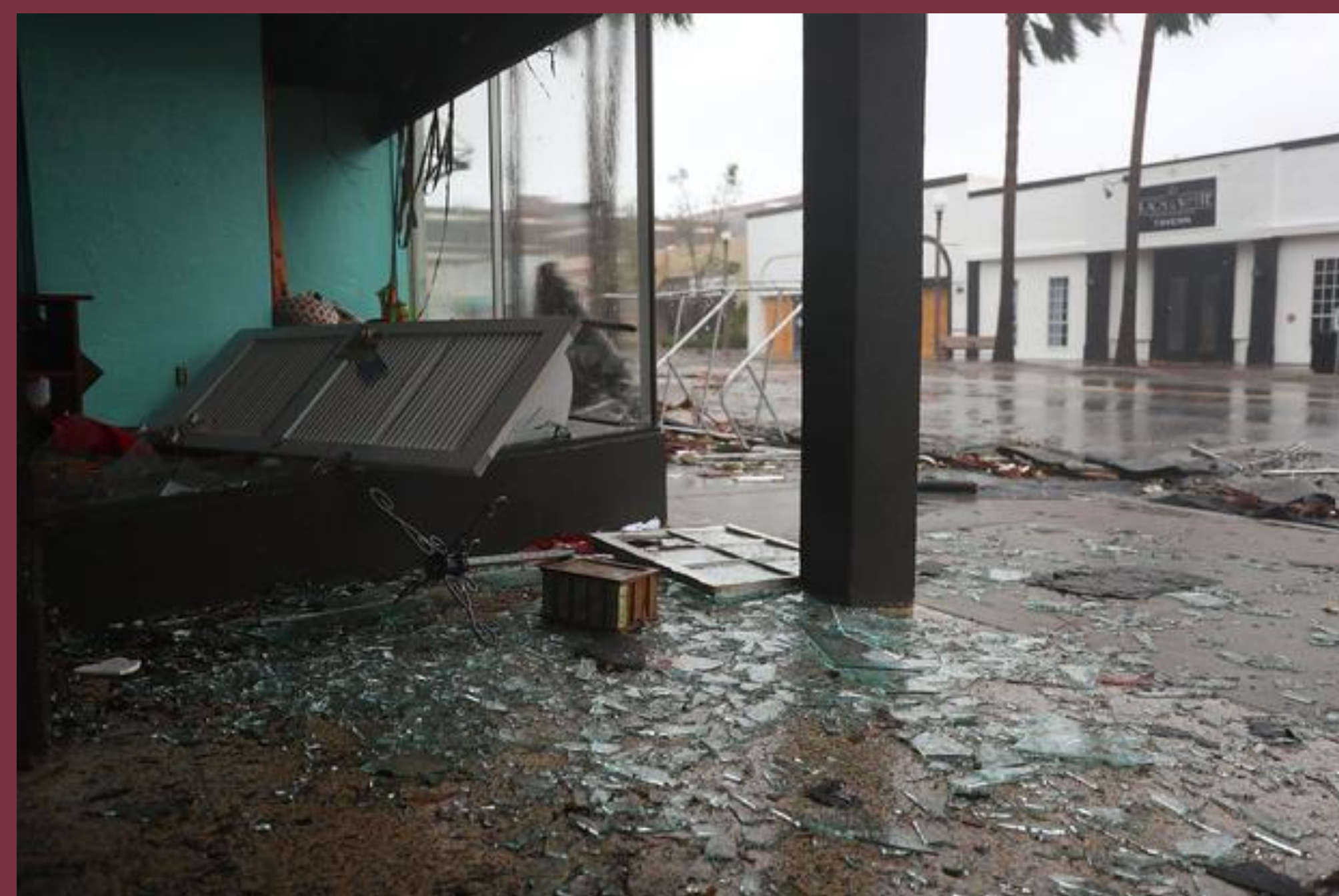
Photo 1. A store in downtown Panama City right after Hurricane Michael.
